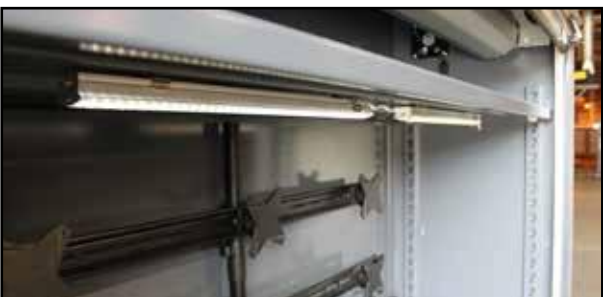
OVERHEAD LIGHTS (LED)
