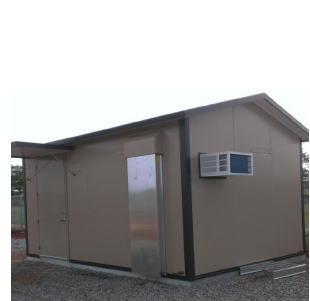
Electric Sub Station
